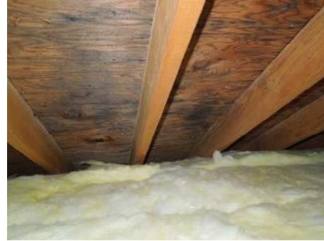
Dark staining at roof sheathing in attic area
