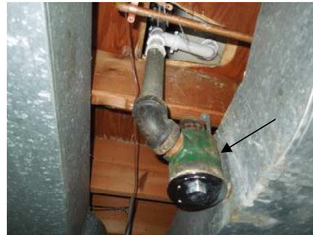
Drum trap at tub/P traps recommended
