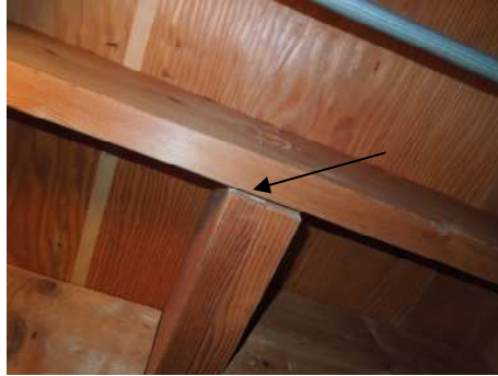
Joist hangers not installed in all recommended areas at basement framing
