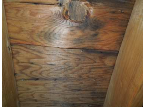
Dark staining at roof sheathing in attic area
