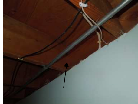
Joist hangers not installed in all recommended areas at basement framing
